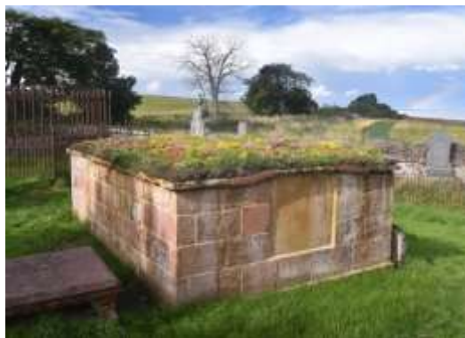
Repair and restoration of the Lady Ardoch tomb, with sedum green roof over a membrane to prevent water ingress
