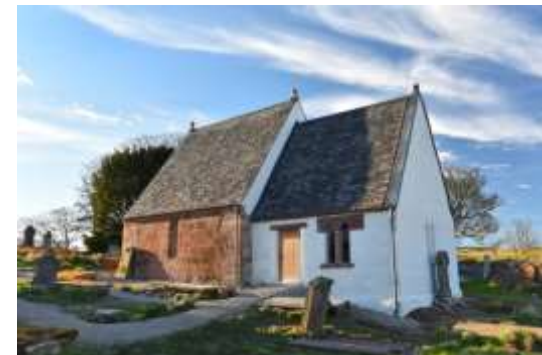
Repair and restoration of the chancel mausoleum
