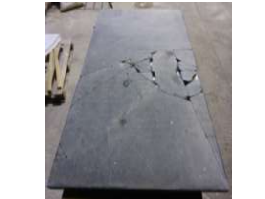
Smashed wall memorial put back in shape before infill with resin and powdered stone to repair
