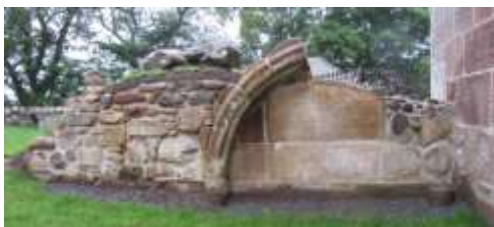
Repair and restoration of the medieval arched tomb recess
